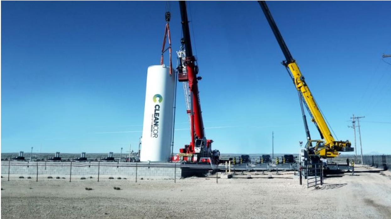
Properly positioning an LNG storage container at a permanent asphalt production facility can be scheduled over a weekend to minimize plant downtime. Photos courtesy of CLEANCOR
